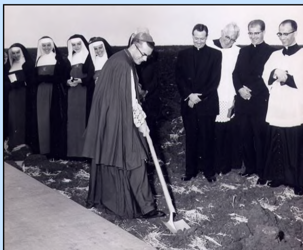
Ground Breaking for Mary & Joseph Retreat Center
